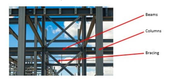
The other common question is what type of building is excluded. This would be a structure, known as frame-built<sup>12</sup> construction where the structure is very repetitive in nature and if one structural element fails, there is not a possibility for
