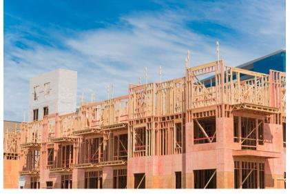
In some cases, there may be a building in which only a portion of it will require inspection. An example of this is shown in the photograph below where the bottom concrete portion of the building incorporates a PLBS as well as a podium deck, but the upper portion is frame-built. In this scenario the bottom will require inspection, but the top will not.
